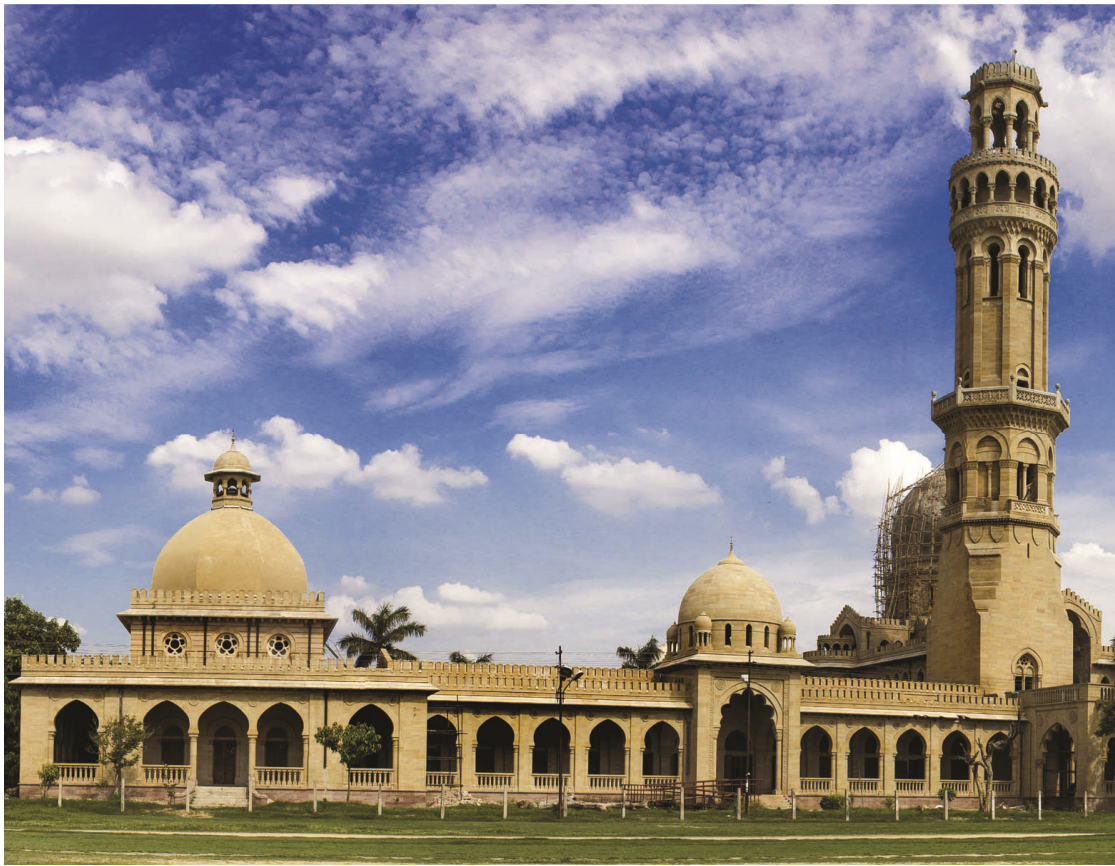
Renovated Vijayanagaram Hall
